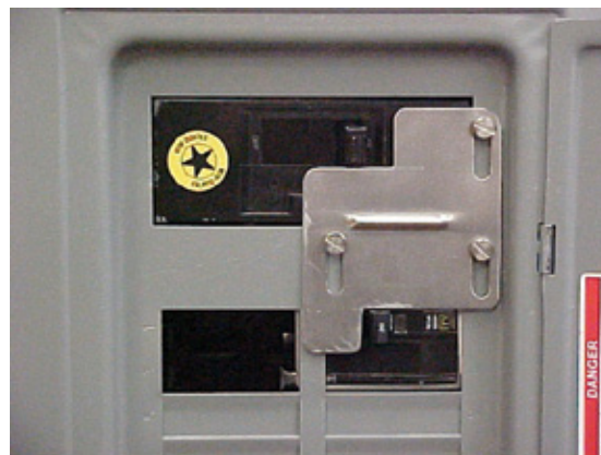
Generator Interlock Kit (In use)
